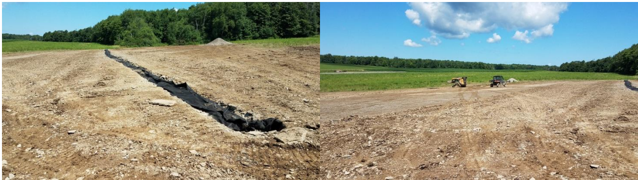
Level Lip Spreader Installation
