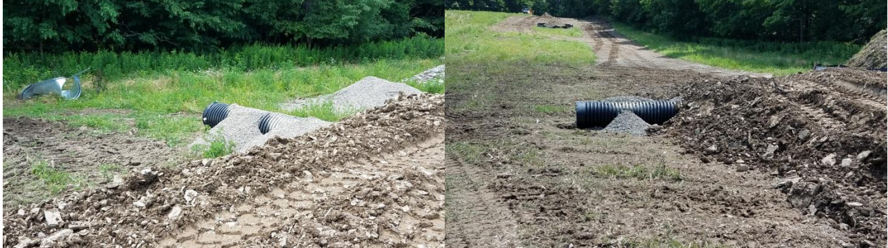
Second Culvert Install
